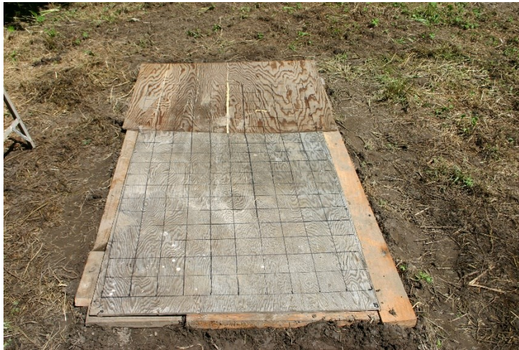
Figure 5: Covering the model with plywood.
